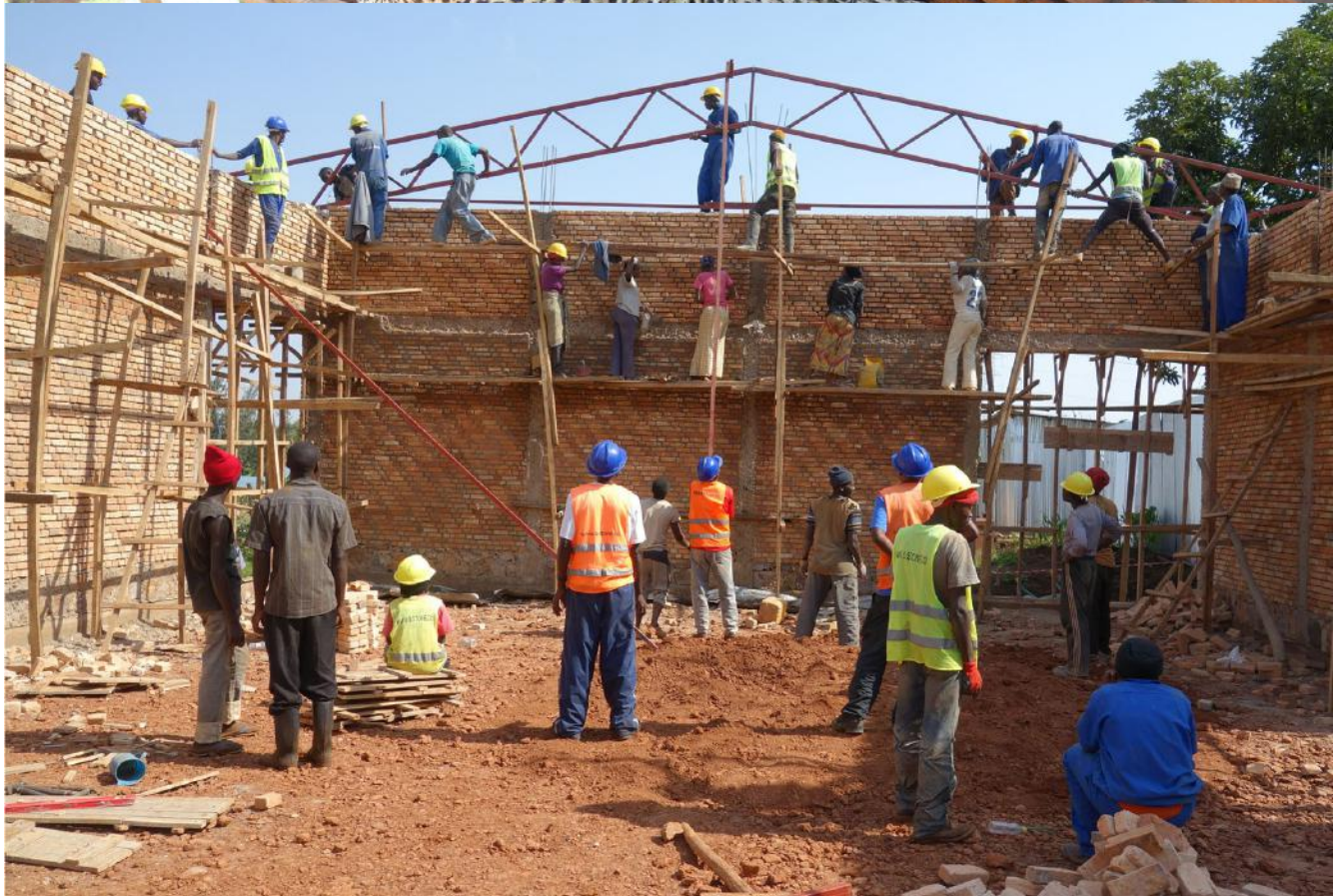
GA Collaborative, Abahizi Dushygikirane Corporation, new building of factory
