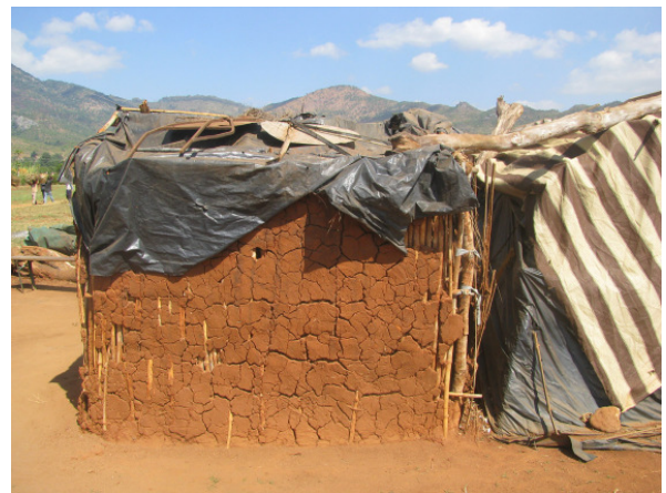
Walls coated with earth in an informal market in Manica, Mozambique. Photo by Paulo Carneiro
