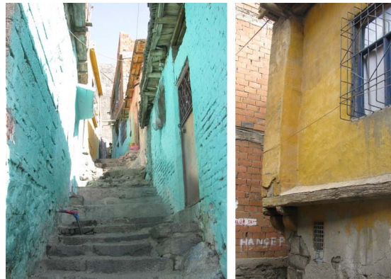
Houses with different colors, Ben-U-Sen in Diyarbakir, Turkey. Photo by Paulo Carneiro
